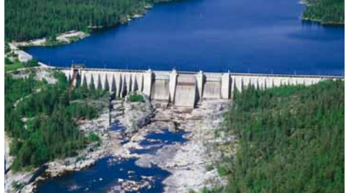
Motor & Generator coolers. Used to cool large electric motors and generators using, for example, river water.
