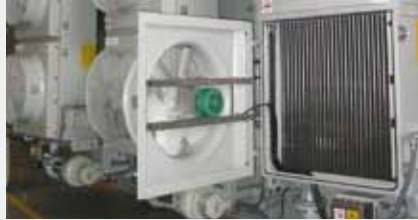
Transformer oil cooler with hinged swing-open fan panels for easy access and cleaning.
