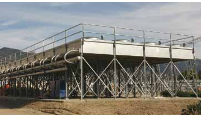
Radiators/Air blast coolers. For watercooling of large diesel engines, chillers for air conditioning, waste incinerators, etc.
