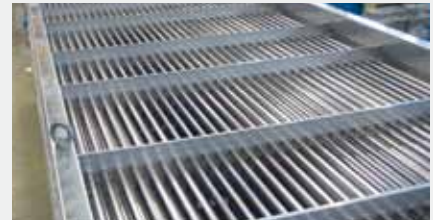
Steel coils QSAK. Finless plain tube design. Used to heat air using heat energy from steam or liquid supplied.
