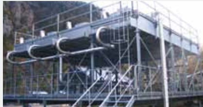
Air blast cooler for application HVDC is used for cooling glycol/pure water with air. The cooling fans are separated from one another by partitions.
